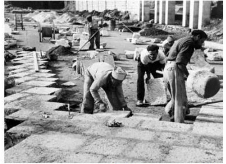
Building a road in Palermo, Italy.
